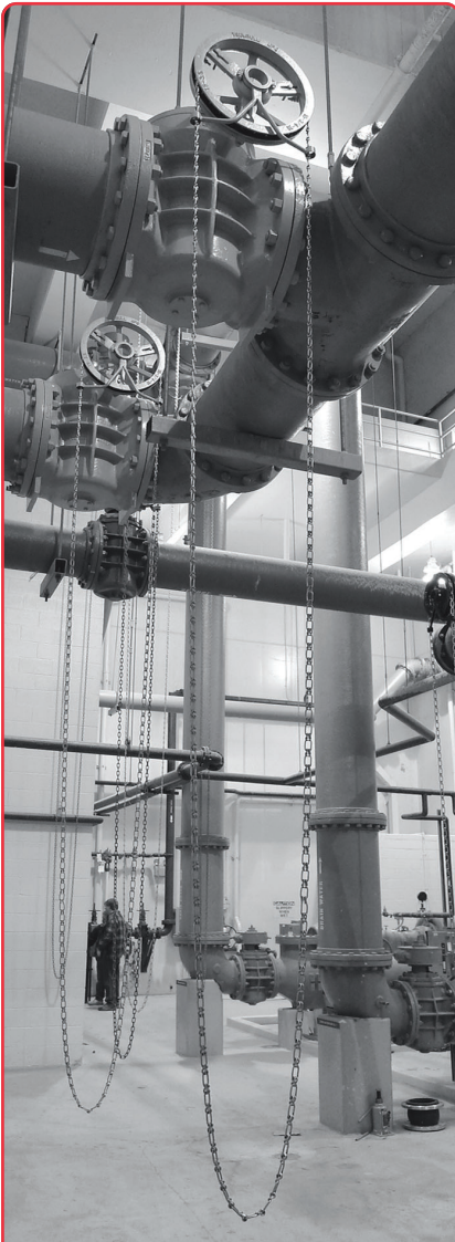
CHAIN FROM OVERHEAD CHAINWHEEL SHOWN IN PATHWAY.
