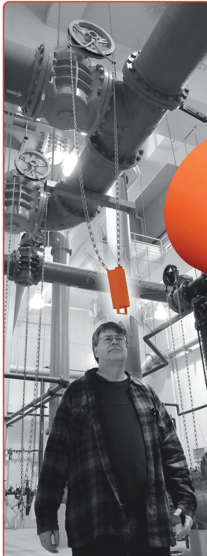
"CHAIN-UP" DEVICE STORES THE CHAIN ABOVE PATHWAY.
