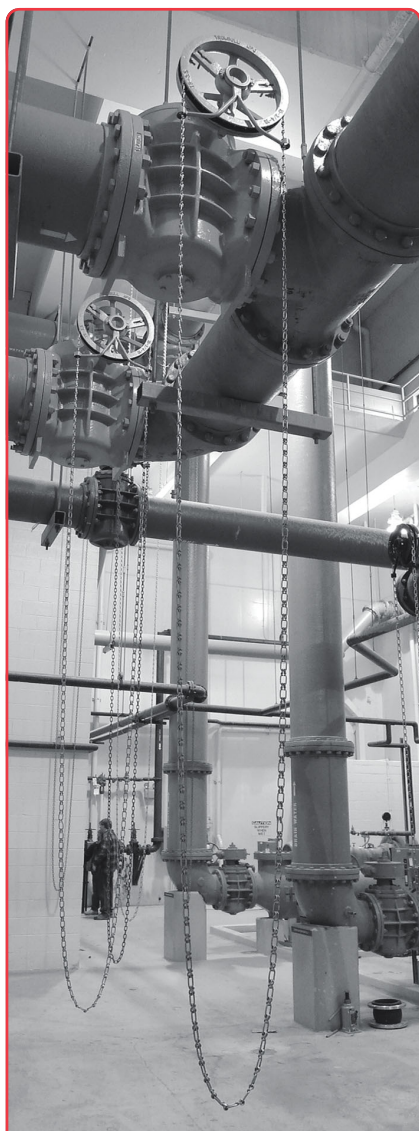
CHAIN FROM OVERHEAD CHAINWHEEL SHOWN IN PATHWAY.
