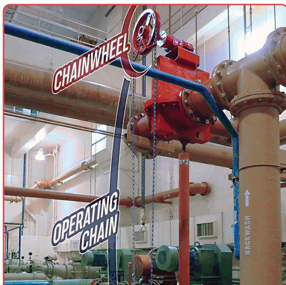
CHAINWHEEL OPERATION ILLUSTRATED.
