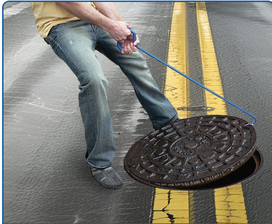
MANHOLE HOOKS ENGAGE PICK HOLES.
