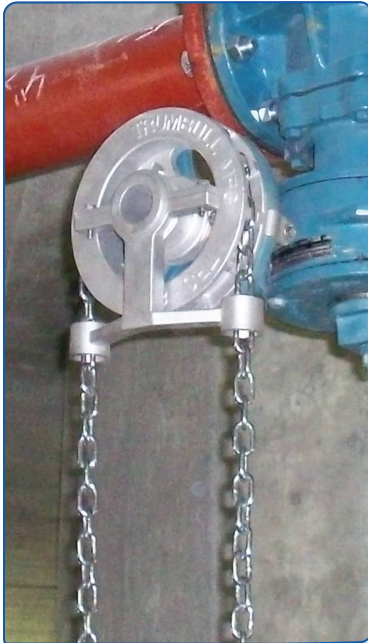
USED TO OPERATE OVERHEAD VALVES FROM THE FLOOR.
