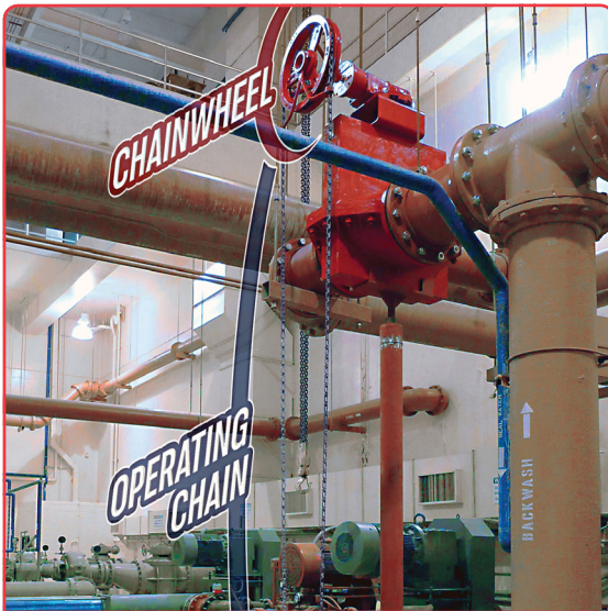
CHAINWHEEL OPERATION ILLUSTRATED.
