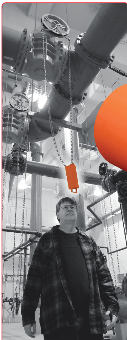
"CHAIN-UP" DEVICE STORES THE CHAIN ABOVE PATHWAY.
