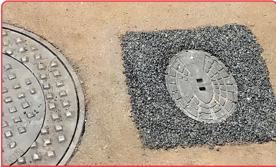
VAULT WITH REMOTE ANTENNA BOX.
