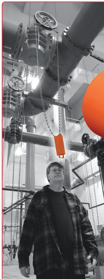
"CHAIN-UP" DEVICE STORES THE CHAIN ABOVE PATHWAY.
