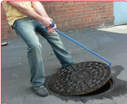
MANHOLE HOOKS ENGAGE PICK HOLES.
