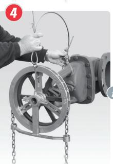
Loop other end of cable around a secure object. Cable can be attached to yoke of valve or an adjacent pipe.
