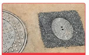
VAULT WITH REMOTE ANTENNA BOX.
