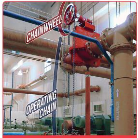
When ordering, indicate the Chainwheel and chain size numbers and the number of feet of chain required. Chain 🦧 is provided in continuous lengths and easily cut in the field to exact length needed. Closing the loop is simple with Connecting Links (shown below), see page G-63 for more information.
