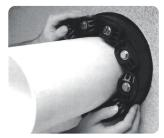
Slide the assembly into the space between the pipe and wall opening.
