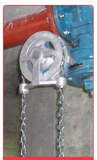
USED TO OPERATE OVERHEAD VALVES FROM THE FLOOR. Stainless Steel Chainwheels allow operation of valves, actuators, or gear boxes in high, hard-to-reach locations by means of a slight pull on the chain. Universal design allows Chainwheel to be clamped to a handwheel, or pinned directly to the stem. Designed for corrosive environments, our Stainless Steel Chainwheels are Type 316 investment steel castings. Ideal in chemical processing, outdoor installations, or salt water environments.
